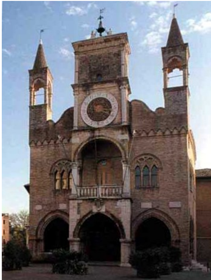
The City Hall Loggia(XIVth cent.) at one end of Corso Vittorio Emanuele
